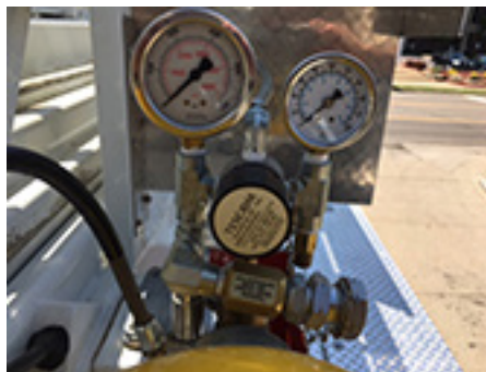
Figure 3-21. Breathing air system gauges
