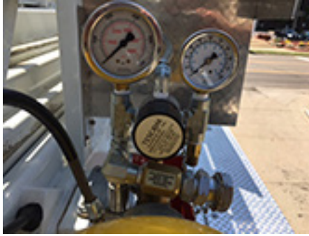
Figure 3-26. Breathing Air System Gauges
