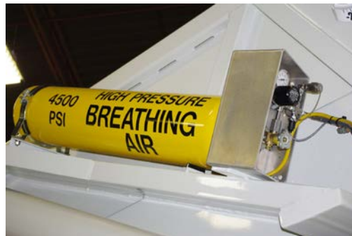
Figure 3-25. Breathing Air System High-Pressure Cylinder
